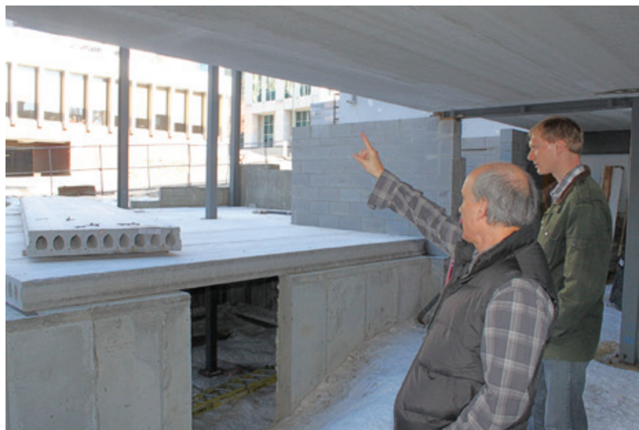
FFRF Co-President Dan Barker and FFRF's newest staff attorney, Sam Grover, look over newly installed floors in Freethought Hall's 9,000 square feet additions.
